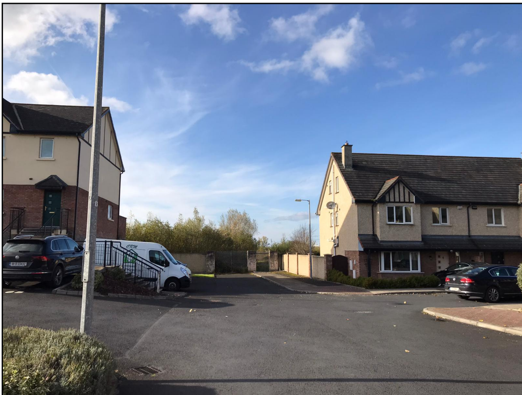
Figure 2.2: Photograph from the Log na gCapall residential estate, showing the existing access gate to the subject lands (TPA, 2020)
